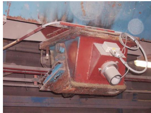
Installation option of the probe in silo outlet with a protective pipe
